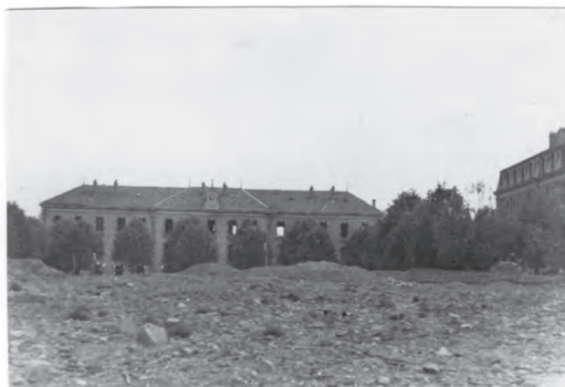
Stalag 315 at Épinal. Destruction seen from the main courtyard, June 26, 1944.
